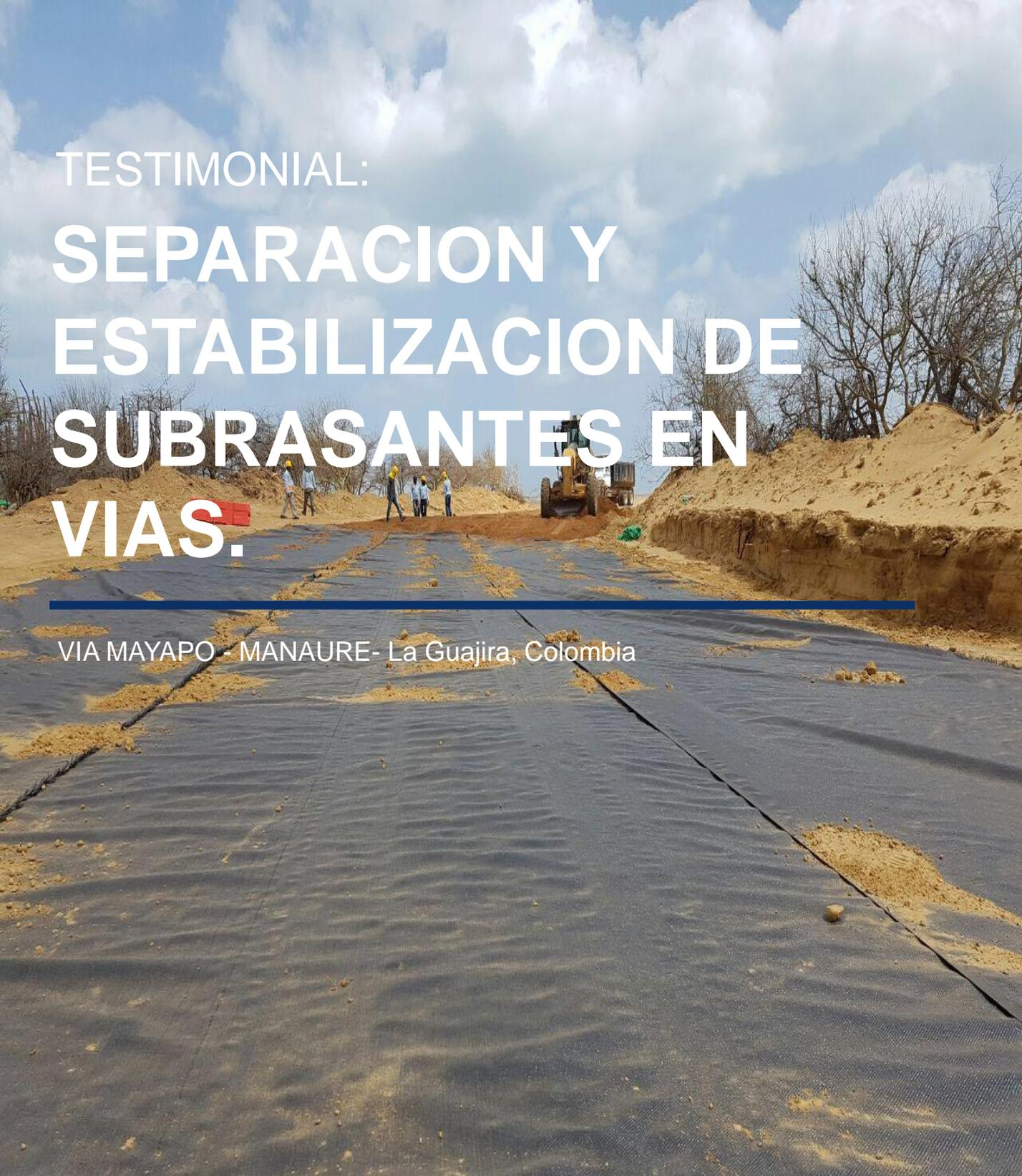
A wide-angle photograph of a construction site. In the foreground, a roadbed is covered with a dark, woven geotextile fabric. Several workers in light blue shirts and yellow hard hats are visible in the middle ground, some standing and others near a yellow excavator. The background shows a dirt embankment and some bare trees under a blue sky with scattered white clouds. The overall scene depicts the process of road stabilization and separation.
